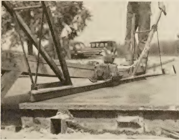
FIGURE 12.—T-BAR AND VIBRATOR USED IN FORMING GROOVES FOR WEAKENED-PLANE JOINTS.
